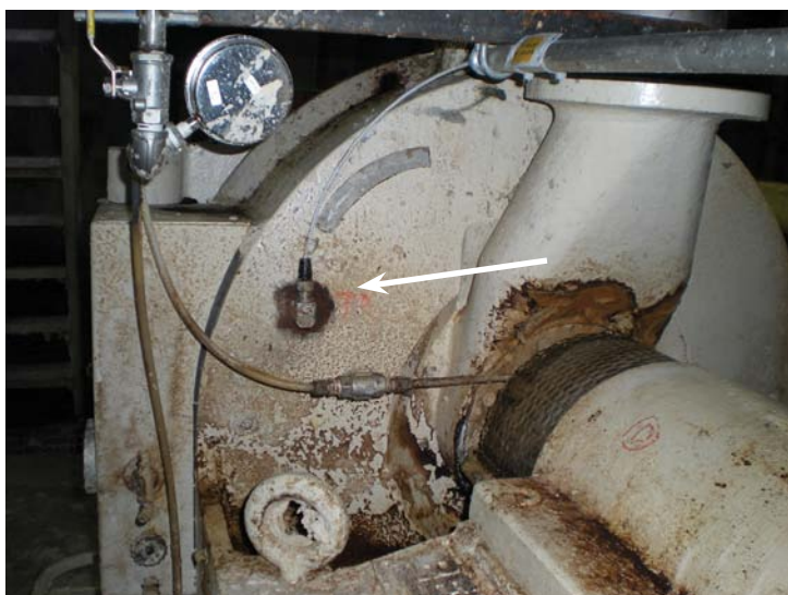
Figure 3 - Mounted Sensor - Outboard Housing
