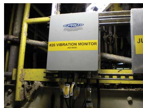
Figure 5 - Junction Box Mounting
