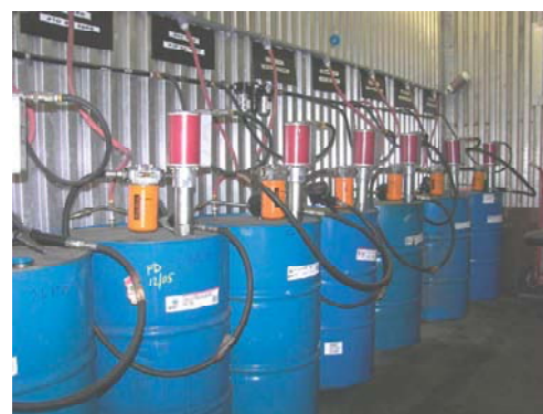
Figure 4. Lube oil room with air pumps and in-line filters for metering heads.
