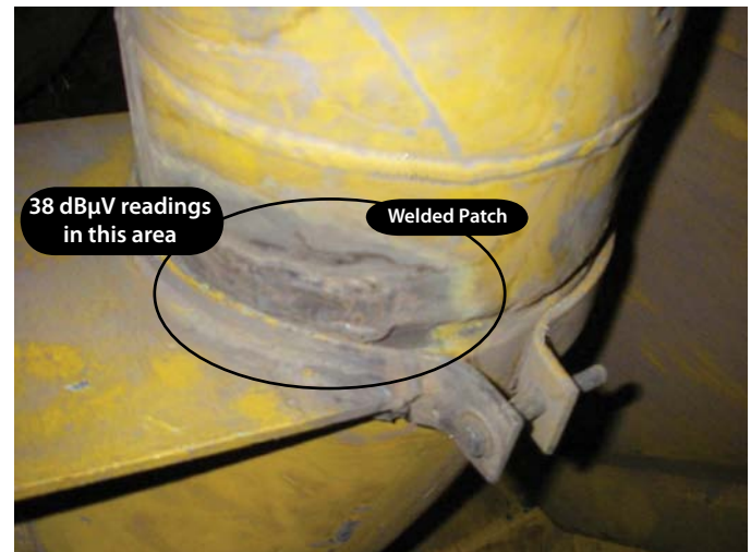
Figure 9 - A leak was discovered where a previous problem had been addressed with a welded patch.
