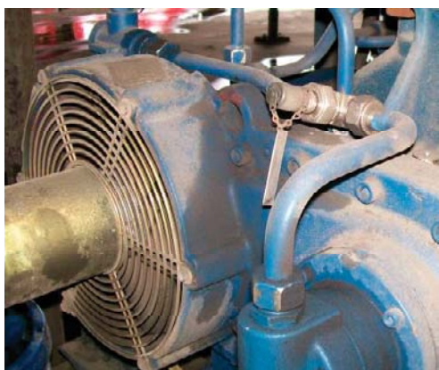
Figure 7 - A good location for a sample fitting to gather oil for testing.
