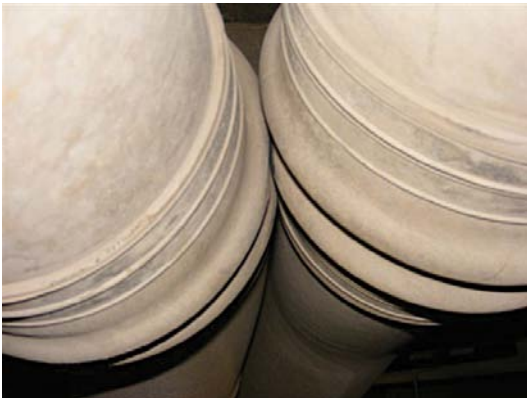
Figure 12 - Breather pipes, which should be at least 1 inch apart, are too close together.
