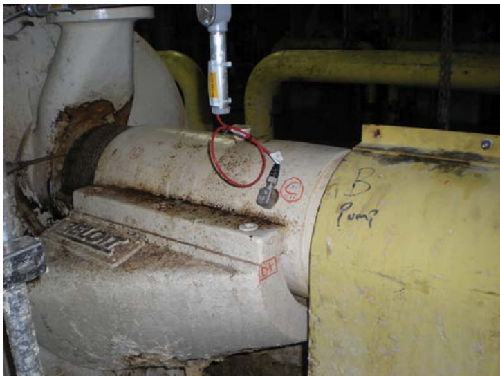
Figure 2 - Sensor Mounting Location - Inboard Bearing
