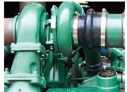
Figure 4 - Typical Turbo Charger System
