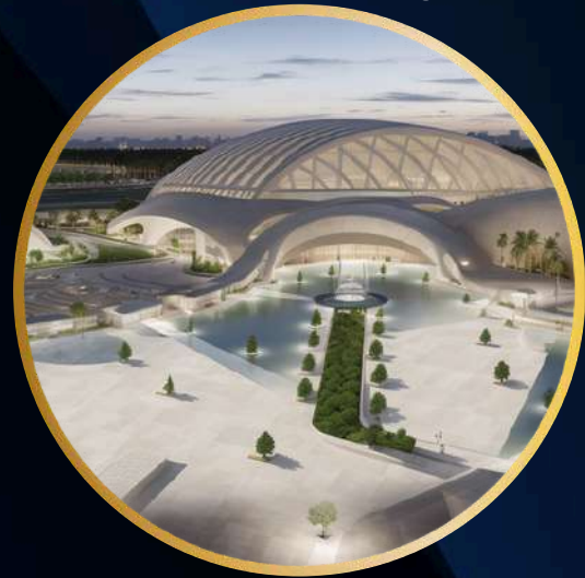
Convention Center, Jeddah (KSA)
