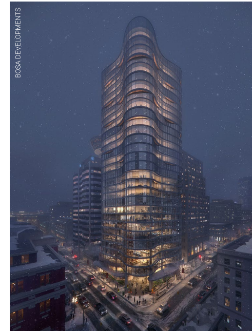
BOSA WATERFRONT CENTRE 320 Granville Estimated Completion Date: Q2 2022 Developer: Bosa Development Square Feet: 374,790
